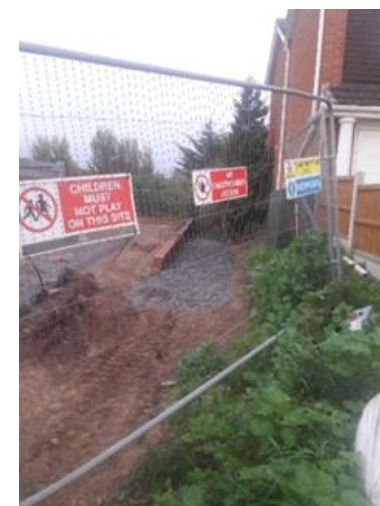
Figure 19- Developer blocking a footpath in Shrewsbury
