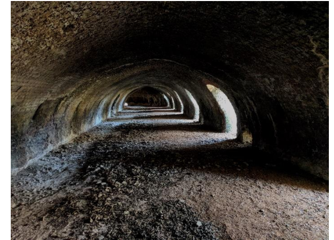
Figure 13- Hoffamn Kiln, Llanymynech Limeworks- A Scheduled Ancient Monument
