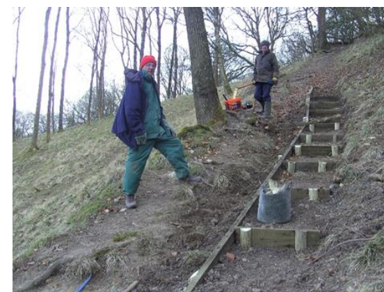
Figure 30- New steps at Gough's Coppice
