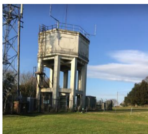
Water Tower (Photo kindly provided by owners)
