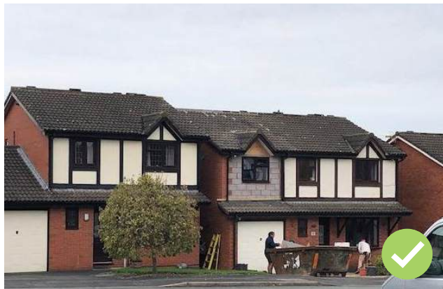
Figure 57: An example of an extension to a property which follows the existing form, scale and materials.
