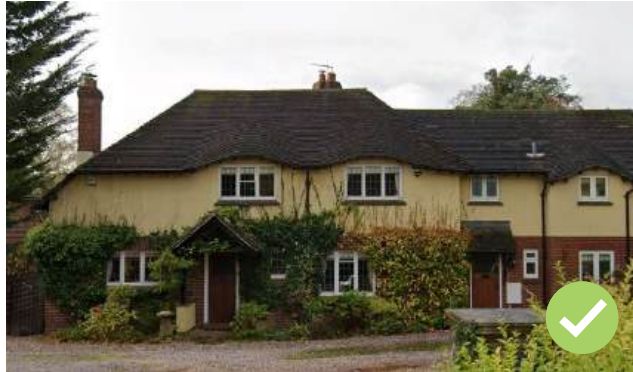
Figure 38: Roofscapes and detailing are varied across the NA. Here, 'eyebrow' detailing along the eave line is a unique arts & crafts style architectural detail.
