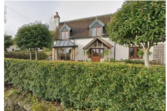
Figure 94: A typical rural cottage as seen in Tasley village.
