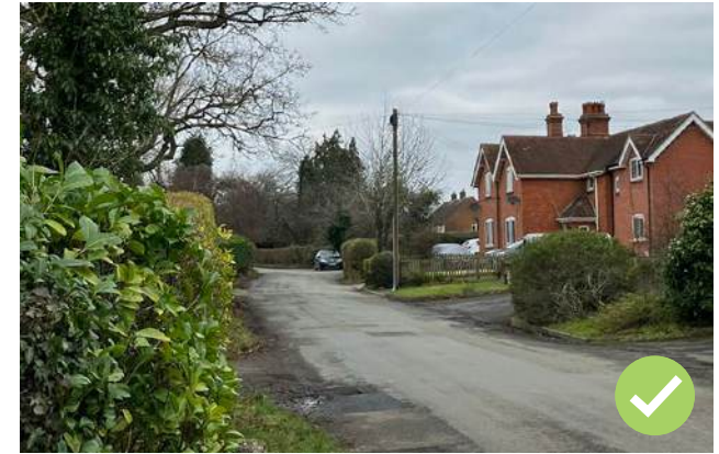
Figure 43: Hedgerows, mature planting, and wooden picket fencing remain common boundary treatments to the south of Church Lane.
