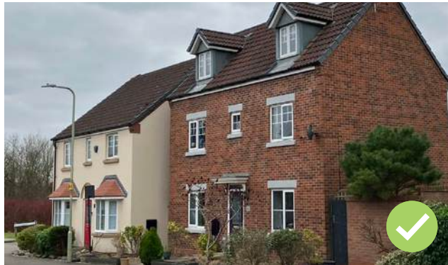
Figure 68: A locally characteristic mix of (multi-tonal) red brick and pale render. Architectural features such as dormer windows sparingly used.
