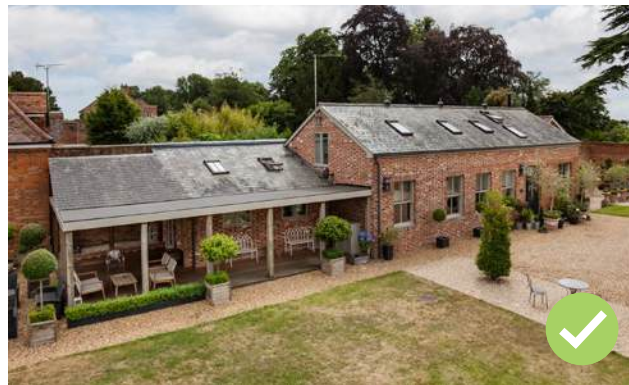
Figure 161: An example of a rural building conversion which complements the existing character.
