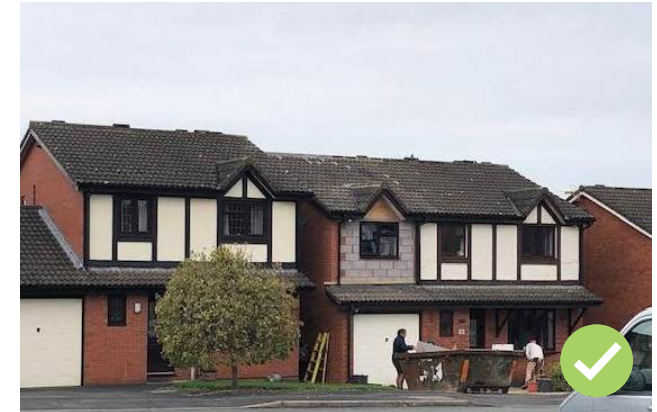
Figure 107: An example of an extension to a property in Tasley which follows the existing form, scale, and materials.
