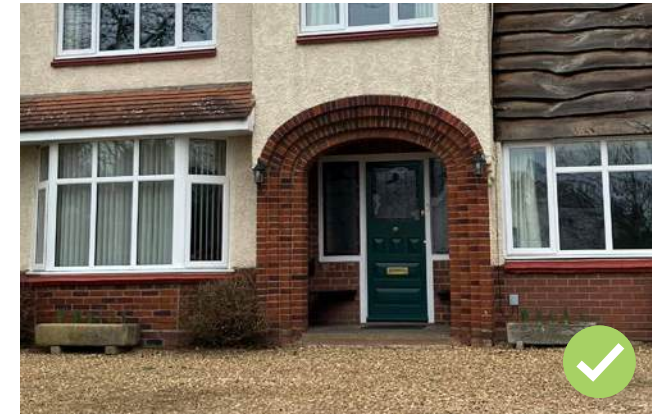
Figure 51: Mainly detached homes with a mix of architectural detailing. A notable recurring feature is arched brickwork detailing around entranceways.
