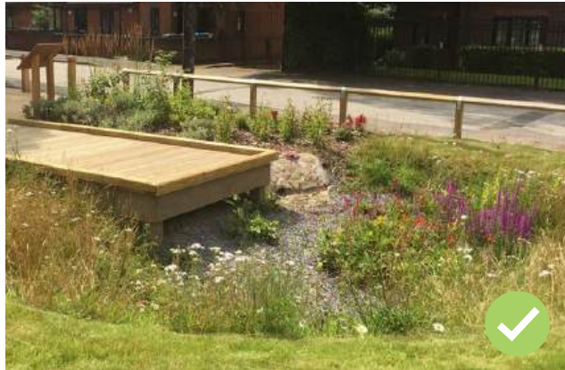
Figure 142: SuDS included within a housing scheme in West Gorton, Manchester.
