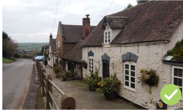
Figure 86: Isolated grouping of buildings are located throughout the countryside. Traditionally 1-2 storeys in height, with variation in orientation and eave/ridge-lines.
