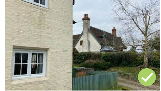
Figure 40: There are a variety of chimney placements and styles on show, including chimney stacks tied to gable ends, as seen here.
