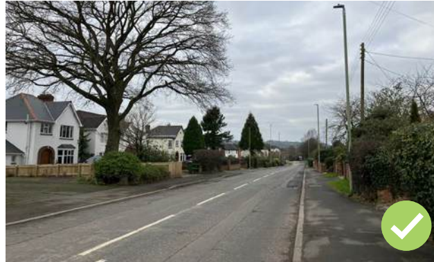
Figure 47: Wenlock Road is a two lane road with footpaths on both sides of the carriageway.
