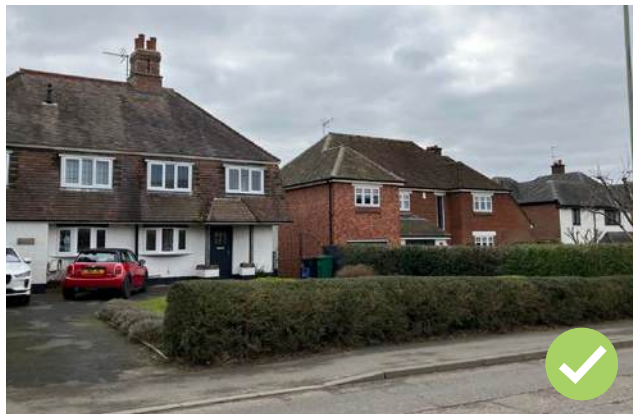
Figure 49: Plot widths and building lines are relatively consistent, which gives a sense of uniformity to the street, despite differences in architectural style.
