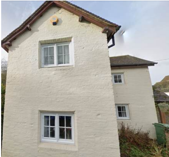
This example shows the use of painted brickwork, cottage style windows, plain clay tiled roof with traditional eaves detail.
