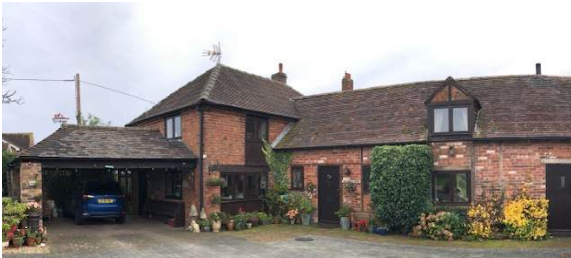
The above shows a converted former barn in traditional handmade soft-red brick, small plain clay tiled steeply pitched roofs, small pitched roofed dormer windows and replacement windows which have kept the traditional vertical emphasis and simple form.
